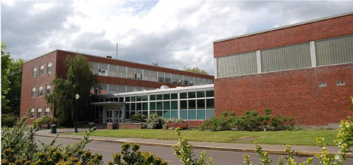
Figure 1 - Photo of the south entrance to Withycombe Hall, pre-renovation.
