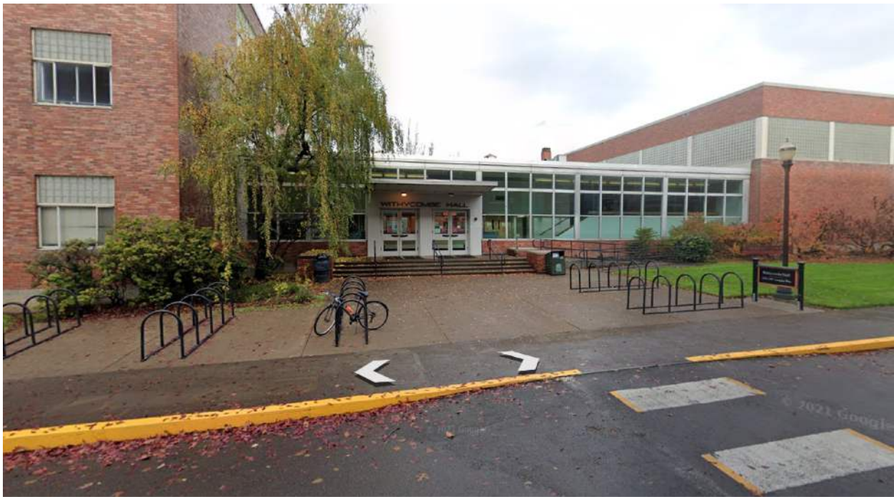
Figure 3 – Google Street-view image of Withycombe Hall's south entrance, pre-renovation.
