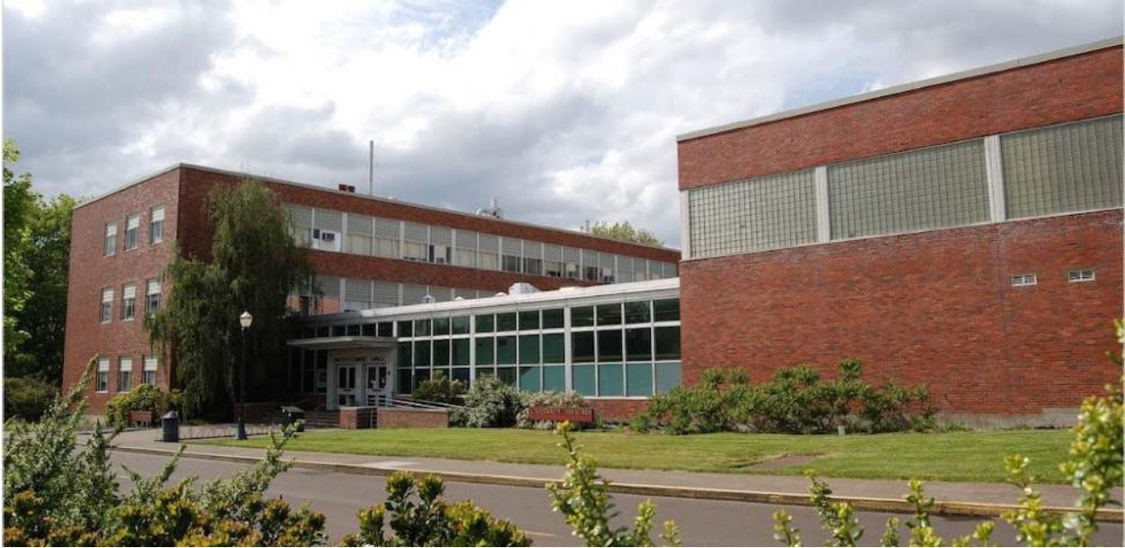
Figure 10 - Photo of Withycombe Hall south entrance prior to renovation.
